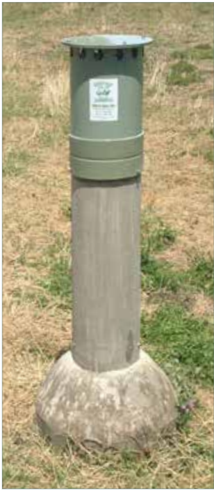
VF300 ON CUT-OFF CONCRETE VENT POLE
