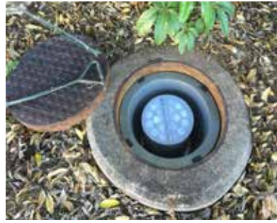
MH300HD MANHOLE ODOUR FILTER
