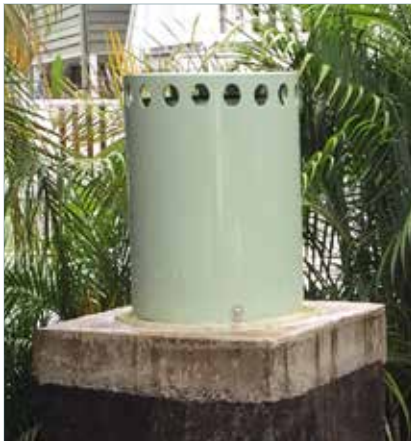
GM300 ON CUT-OFF CONCRETE VENT POLE
